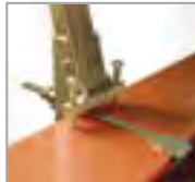
Stanchion installation complete
