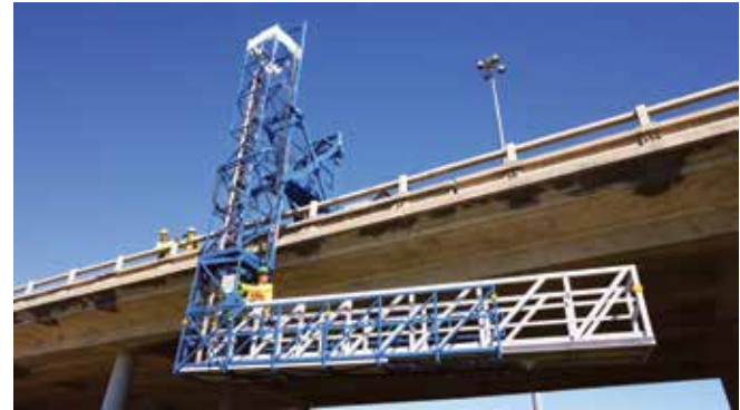
Suspended access hydra platform.
